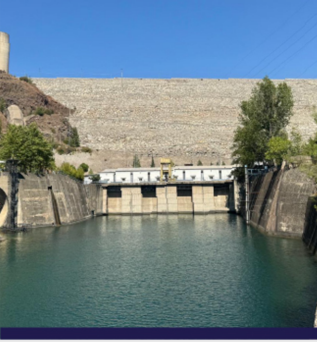
HES ve Baraj Ekipmanları Hydroelectric Power Plant and Dam Equipment
