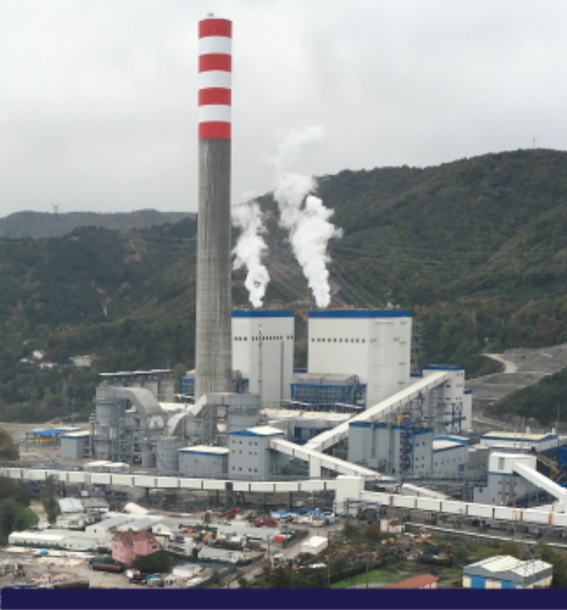
Enerji Santralleri Power Plants
